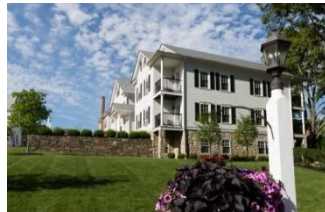
Chamberlain House 20 Guest Rooms
